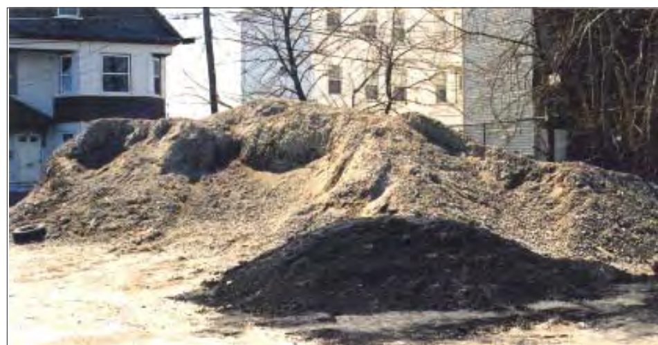
According to neighbors, these piles of landfills and asphalt were dumped during the reconstruction of Broadway.
