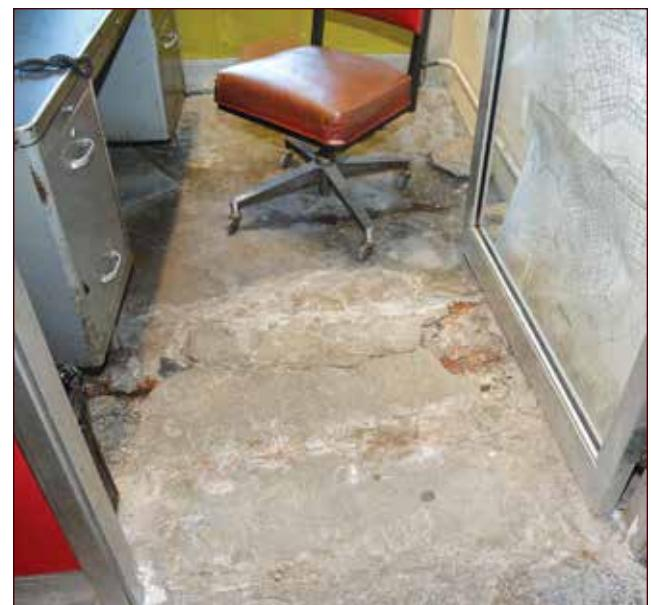
The concrete was lifted by the support installed in the basement, Now the door cannot be closed.
