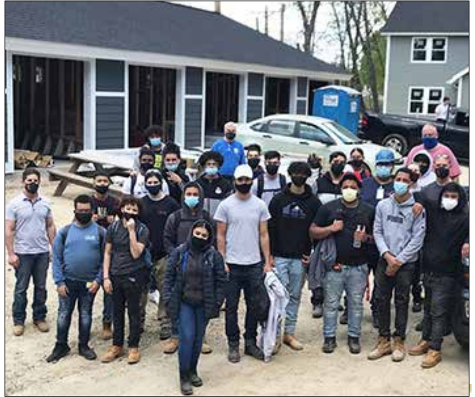
Greater Lawrence Tech carpentry, HVAC, electrical, and plumbing students all worked on the project this year.
